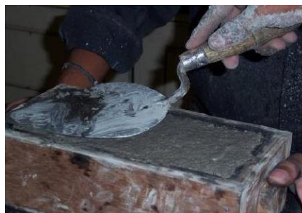
Figure 2: Casting of Bricks
